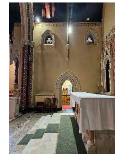
View of door G-D03 to the sacristy, including high level windows W-FO1-02. Plaster finish in this area has a lined-and-ruled finish which differs from the other areas of the church.
