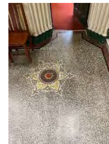
Decorative terrazo and mosaic flooring to alter including door G-D03, in good condition.
