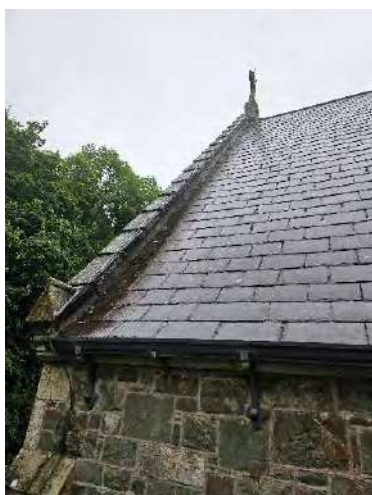
High level roof, north-east end. Slatework, cast iron gutter & brackets and capping detail to wall Roof A, pitch A7.
