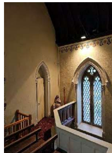
View to the rhs at balcony level including door F-D01 to the bell tower.
