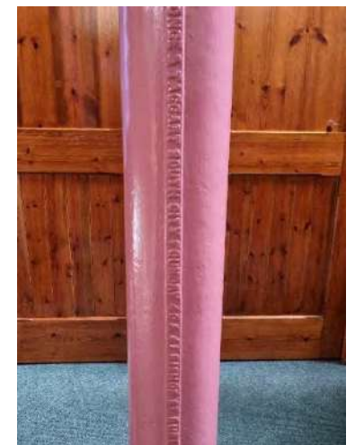
Detail of the cast iron columns supporting the choir balcony "Tonge & Taggart South City Foundry 40 & 41 Bishop St Dublin".
