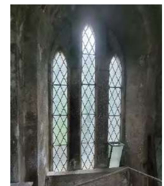
Fig 19: Existing window in belltower with openable section to lower section of window
