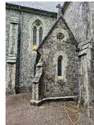
Window W-G11 north east porch. Tarmac surface throughout.
