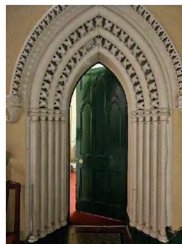
Decorative plasterwork surround detail to door G-DO3 to the sacristy.
