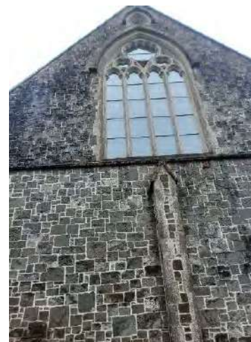
North elevation behind Altar: central. Façade re-pointed. Stained glass window with secondary storm glazing externally.
