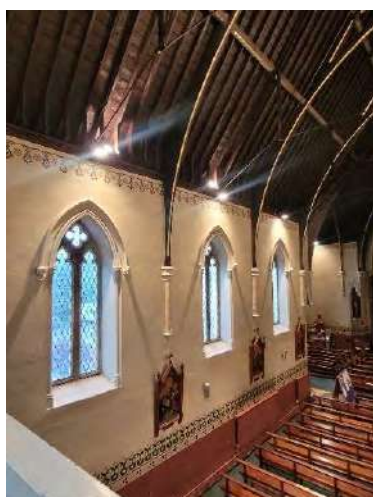
View from the choir balcony to the south of windows W-G20-22, all fixed windows.
