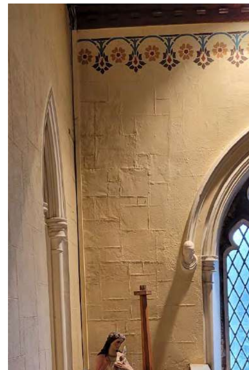
Fig 7: Internal Wall finish with random ashlar pattern and decorative stencilling
