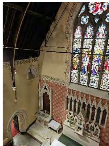
High level view of the alter lhs. Condition of stained glass window not assessed.
