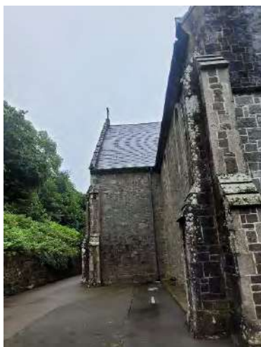
East transept; north elevation. Tarmac surface throughout with small concrete plinth to east wall of Altar.
