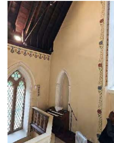
View to the lhs at balcony level including a niche mirroring the plasterwork detail of the door on the opposite side of the balcony. Random ashlar pattern finish with stencilling detail to window.
