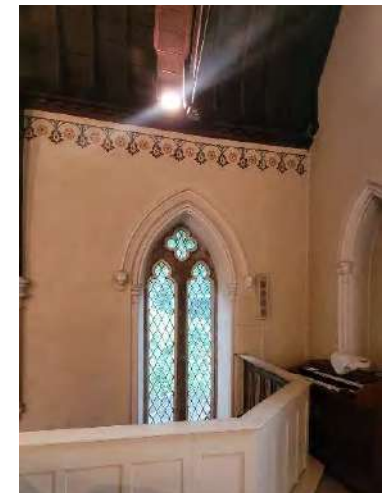
View from the choir balcony of windows W-G15, fixed window. Decorative paintwork stencilling at high level of wall.
