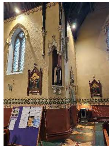
View of corner intersection between windows W-G21 and door G-D12 featuring a high level statue niche, boasted plaster below.
