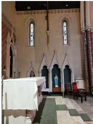
View east of the altar, including windows W-G06-07 at high level and decorative statue niches. Lined-and-ruled plaster finish which differs from the main areas of the church.
