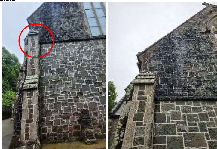
North elevation behind Altar; left hand side. This elevation has been re-pointed circa. 2010, perhaps in two phases, upper and lower.
