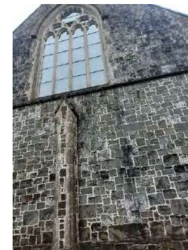
North elevation behind Altar: central. Façade re-pointed.
