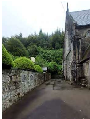
Site boundary wall to north end of church, boundary wall adjoining presbytery. Tarmac surface throughout.
