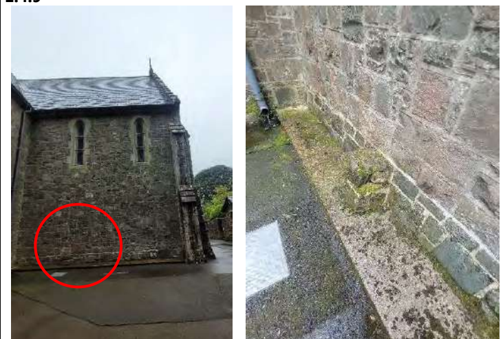
Concrete plinth at base of the wall with a wall nib, possible service area. Base of wall, lower courses, appears to be re-pointed recently.
