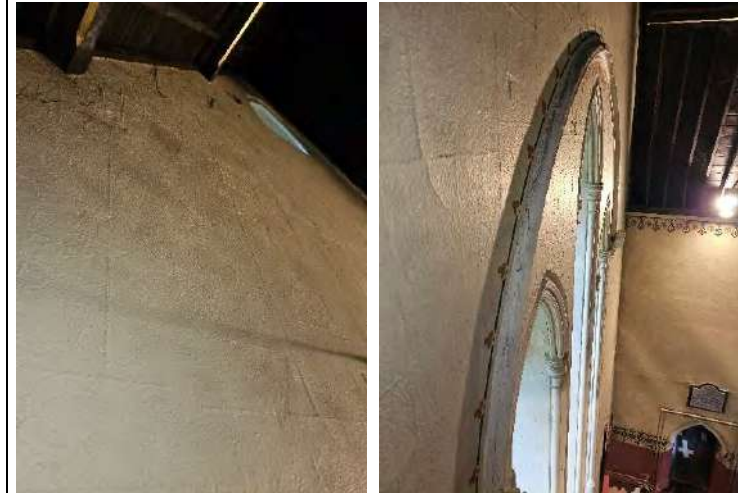
High level view above central window W-G08-10. Note plasterwork and paint finish in fair condition.
