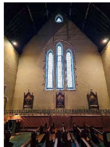
View centrally of west transept including windows W-G24-26. Note boasted plaster below cill level. Opening section to central window, not operational.
