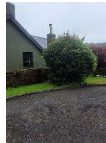
South-west boundary wall, adjoining property beyond.
