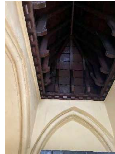
Ceiling view of timber structure, painted dark.
