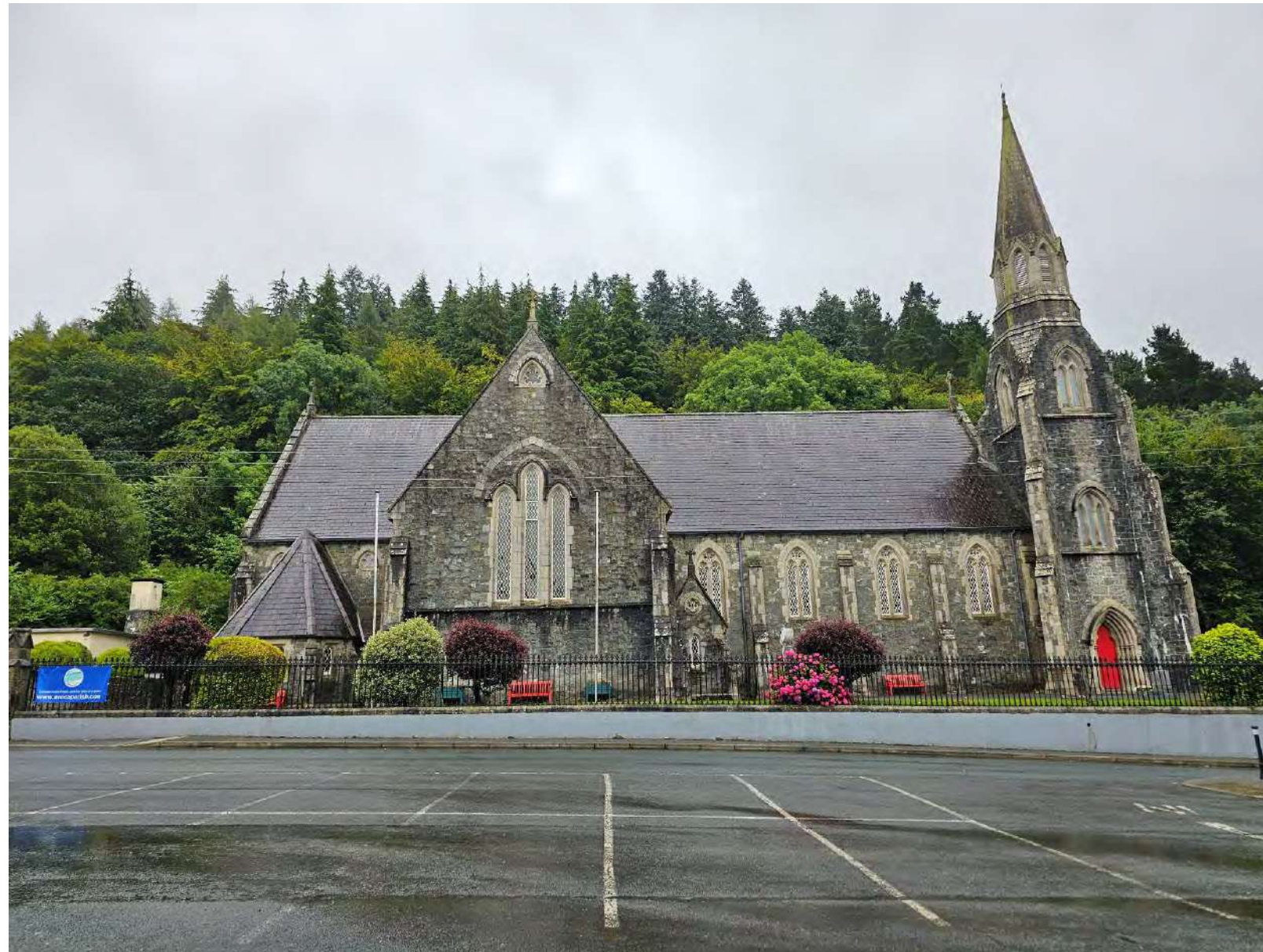
Front Elevation – FKP photo from July 2023
