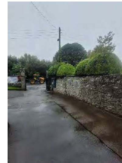
Entrance gates and boundary wall to the north west of the site. Tarmac surface throughout.
