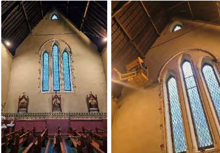
View of east transept. Random ashlar pattern to plasterwork at high level and flat finish to low level. Opening section to central window not operational.
