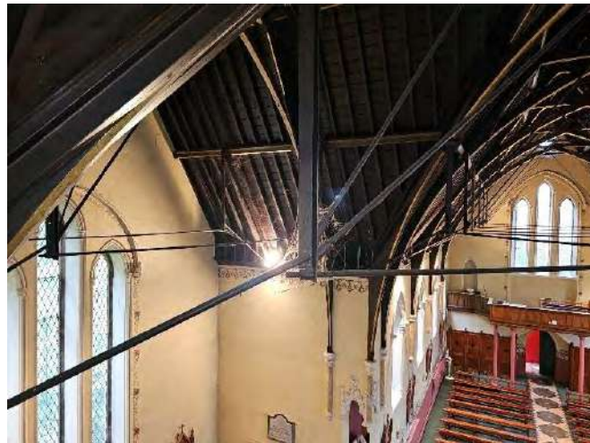
High level view of the roof structure looking south east along the east transept with secondary steel ties apparent.
