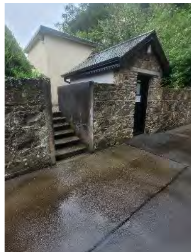
Steps to the Parochial House and parishoner WC to the north boundary wall.
