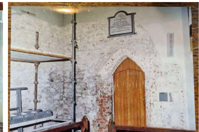
Fig 15: Internal photo of Avoca Church, internal plaster repair work to East Transept, assumed 2000, provided by Fr Michal Murphy P.P.
