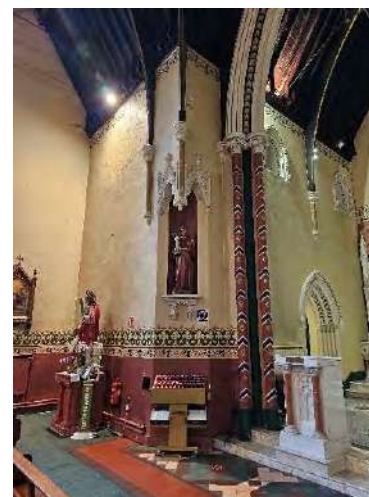
View of corner intersection between west transept and alter area. Windows, featuring a high level statue niche, boasted plaster below.
