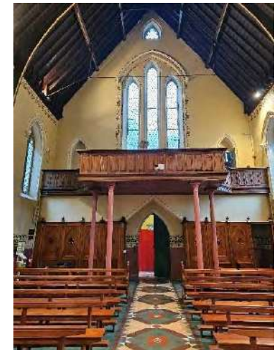
View of central aisle to the south, with choir balcony structure atop cast iron columns, understood to be original to the church.
