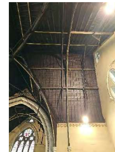
View of the timber roof structure to the east transept.
