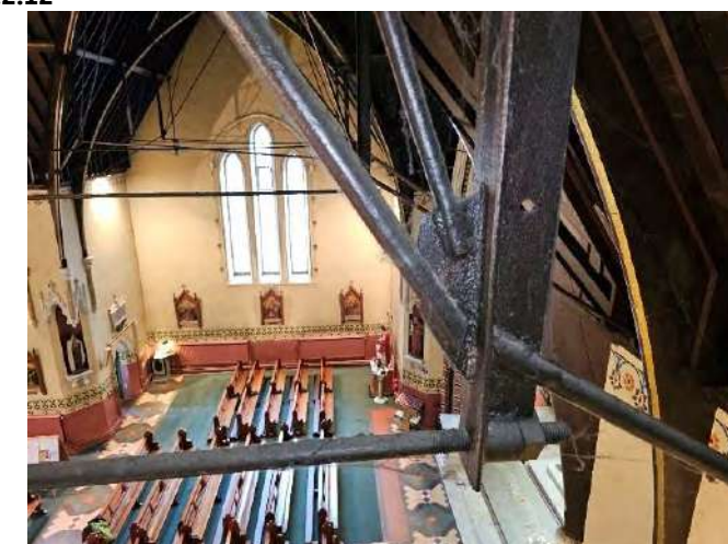
High level view of the west transept including secondary modern steel roof ties.
